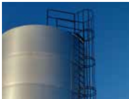
Ladder Safety Caging / Roof Handrail
