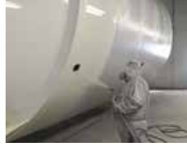
Polyurethane Exterior Coating
