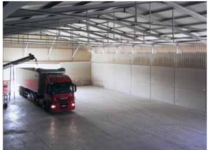
> Storage on removal cart
